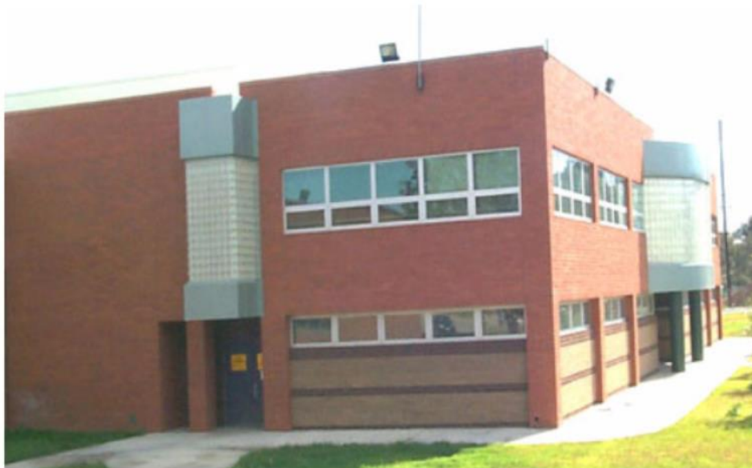
Figure 18. Exterior view of modern reinforced brick masonry building at Roosevelt Elementary School
