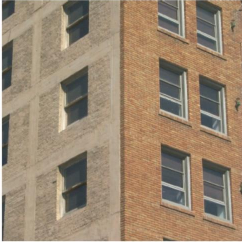
Figure 14. Close-up view of 3711 Roxbury Street building showing exterior infill frame construction
