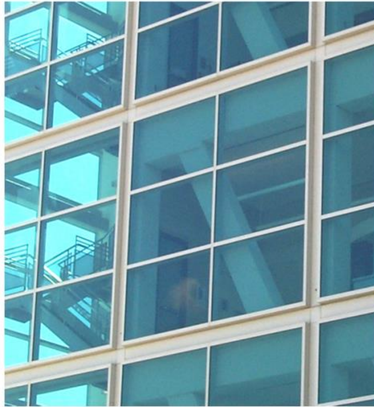
Figure 11. Close-up view of 3703 Roxbury Street exterior showing perimeter braced steel framing.
